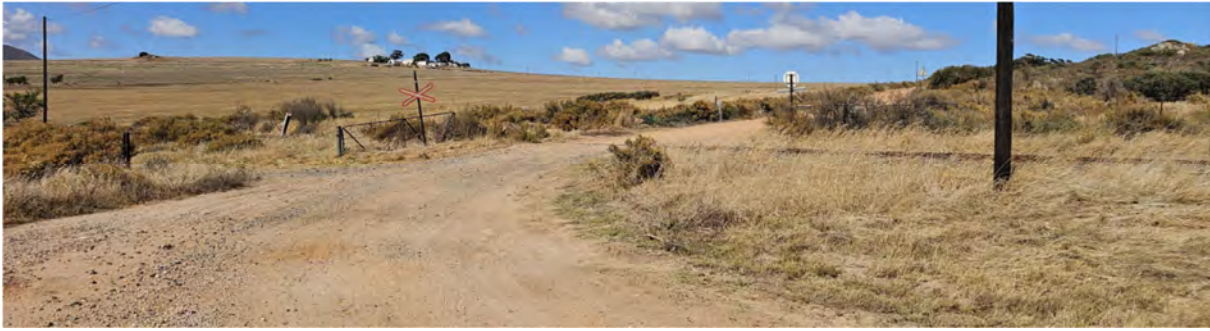
Figure 9: OP5339 railway crossing
